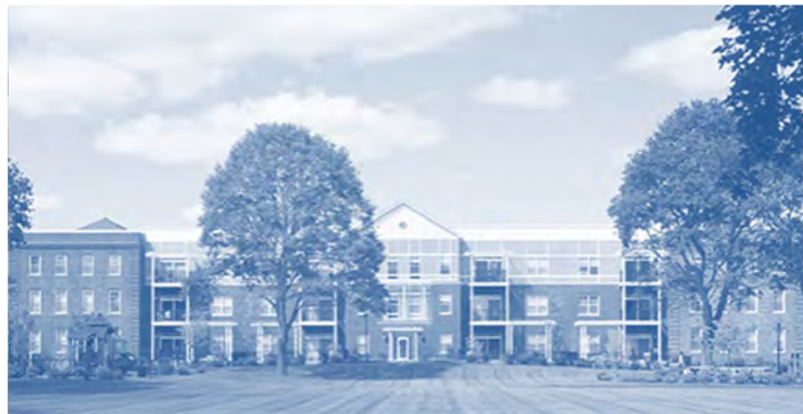
Metropolitan State Hospital Reuse (Waltham/Lexington, Lexington Hills)
